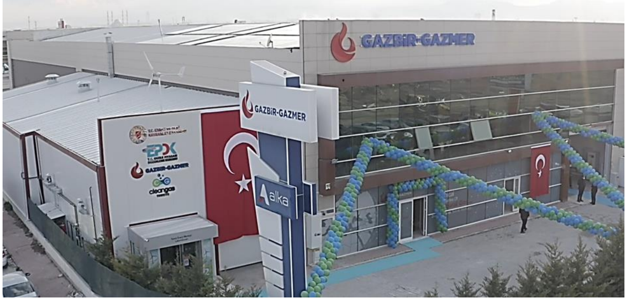
Figure 1.1: Outside view of the Clean Energy Technologies Center.
